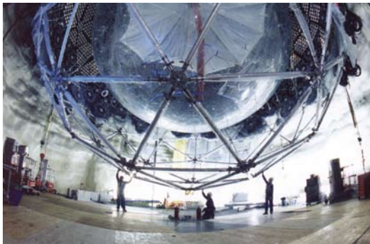
SNO detector during construction
